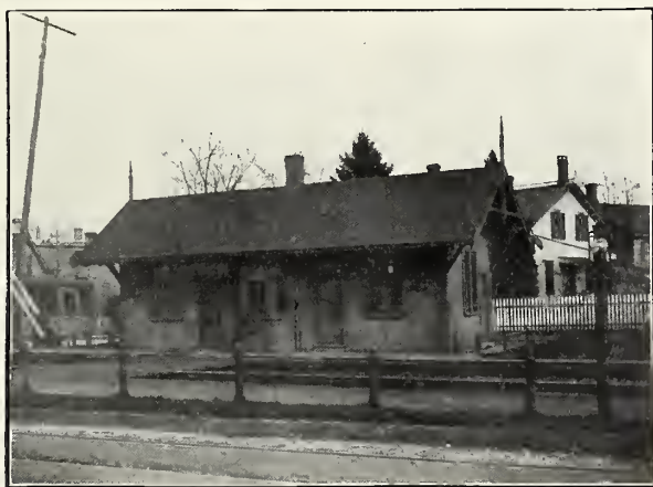
THE PROSPECT STREET DEPOT.
